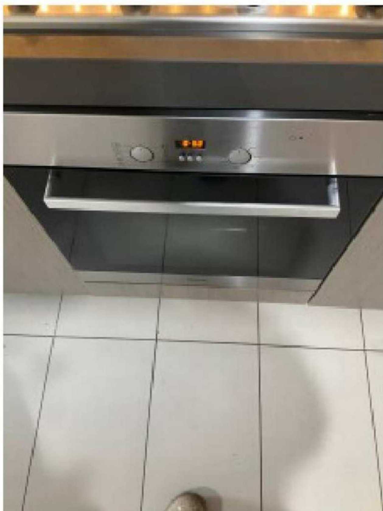
Oven is tested and operational at the time of inspection
