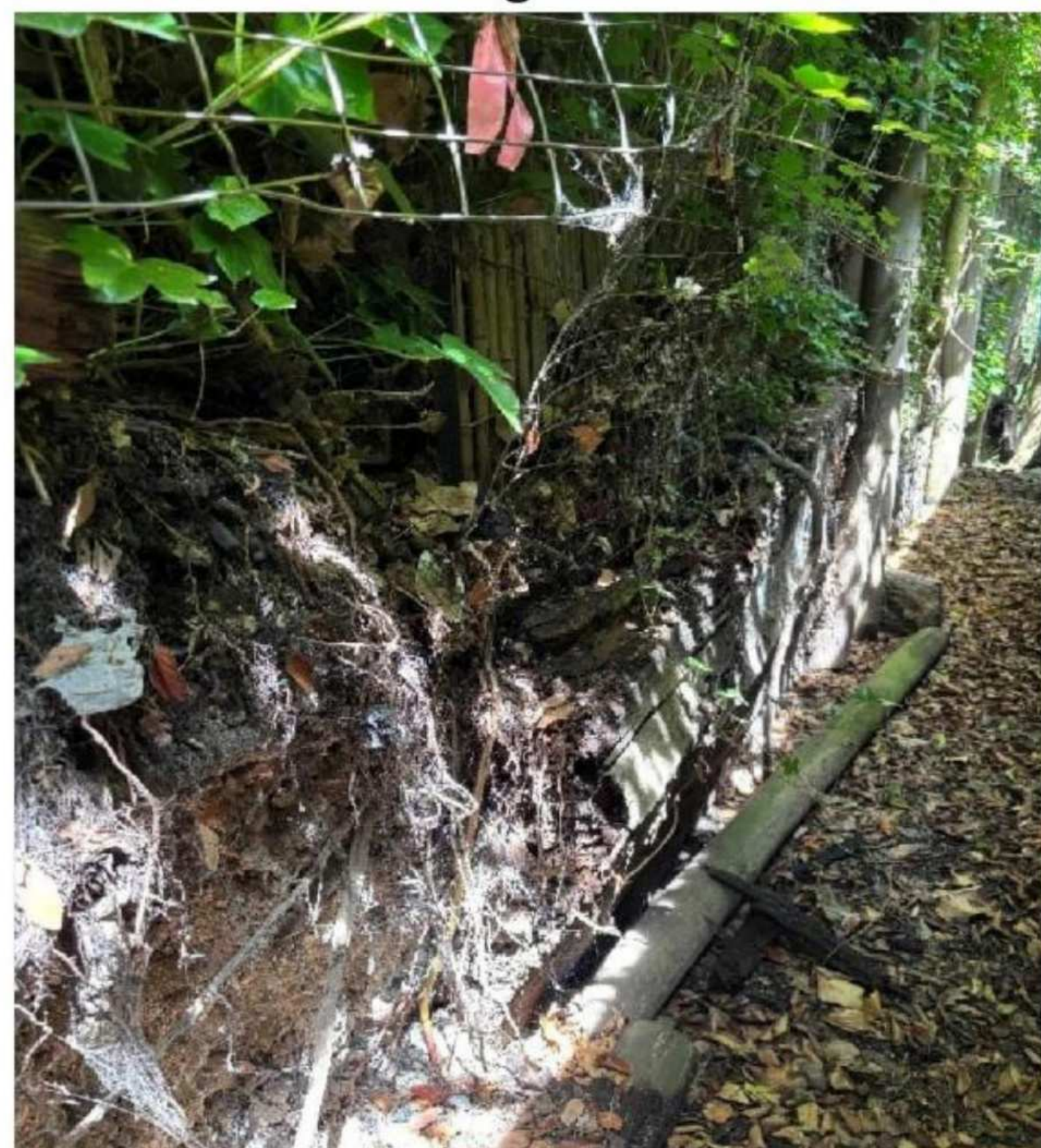
South side retaining wall
