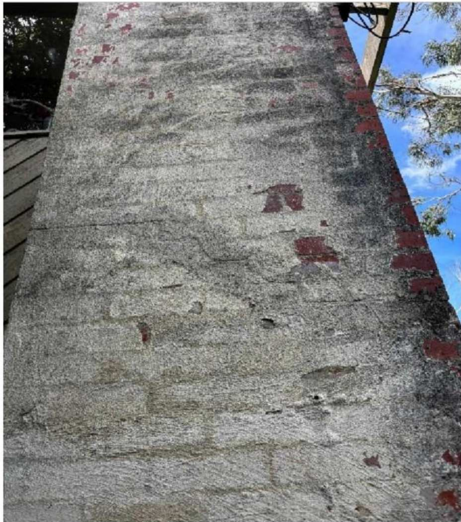
North west corner
