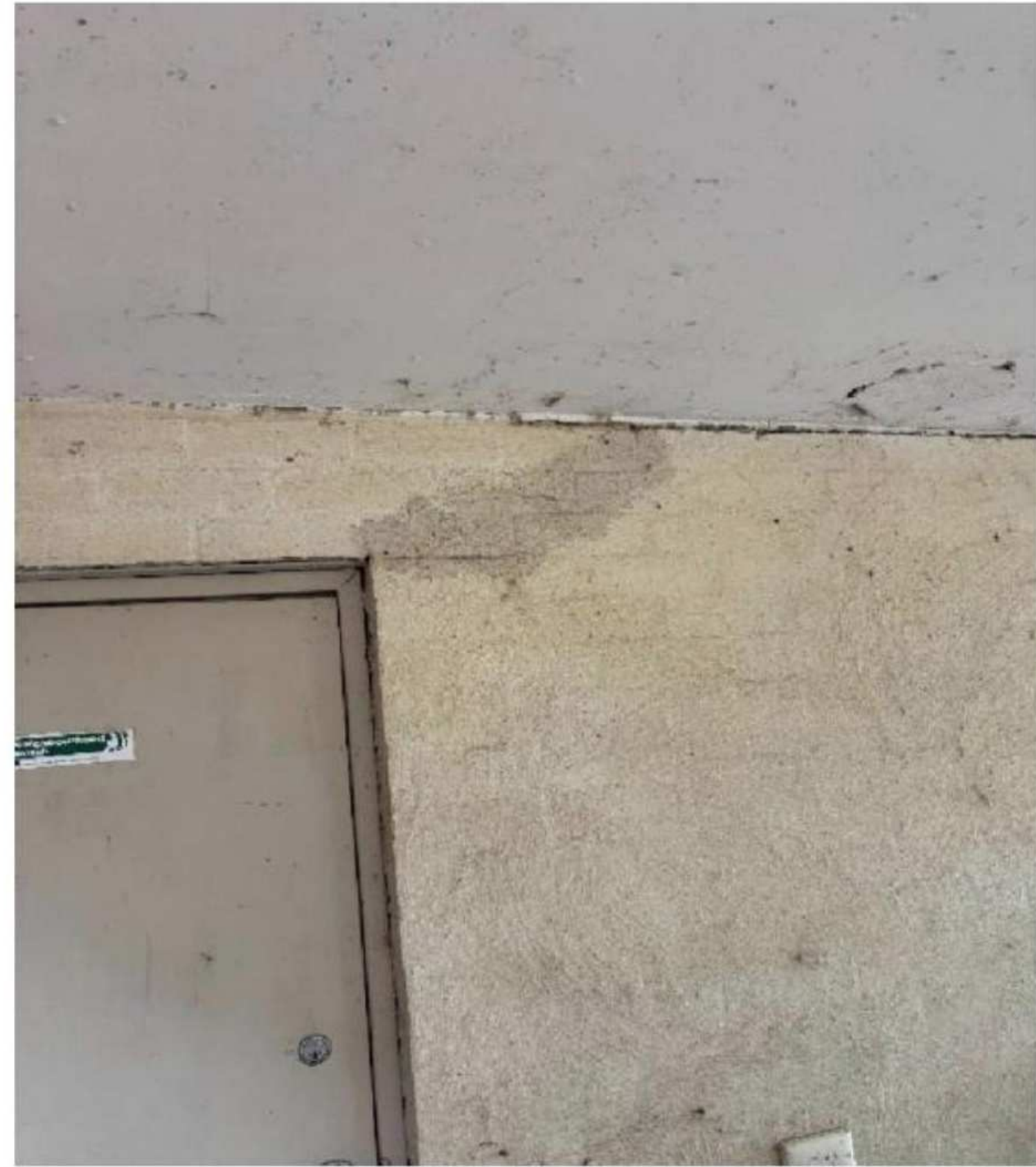
North west corner
