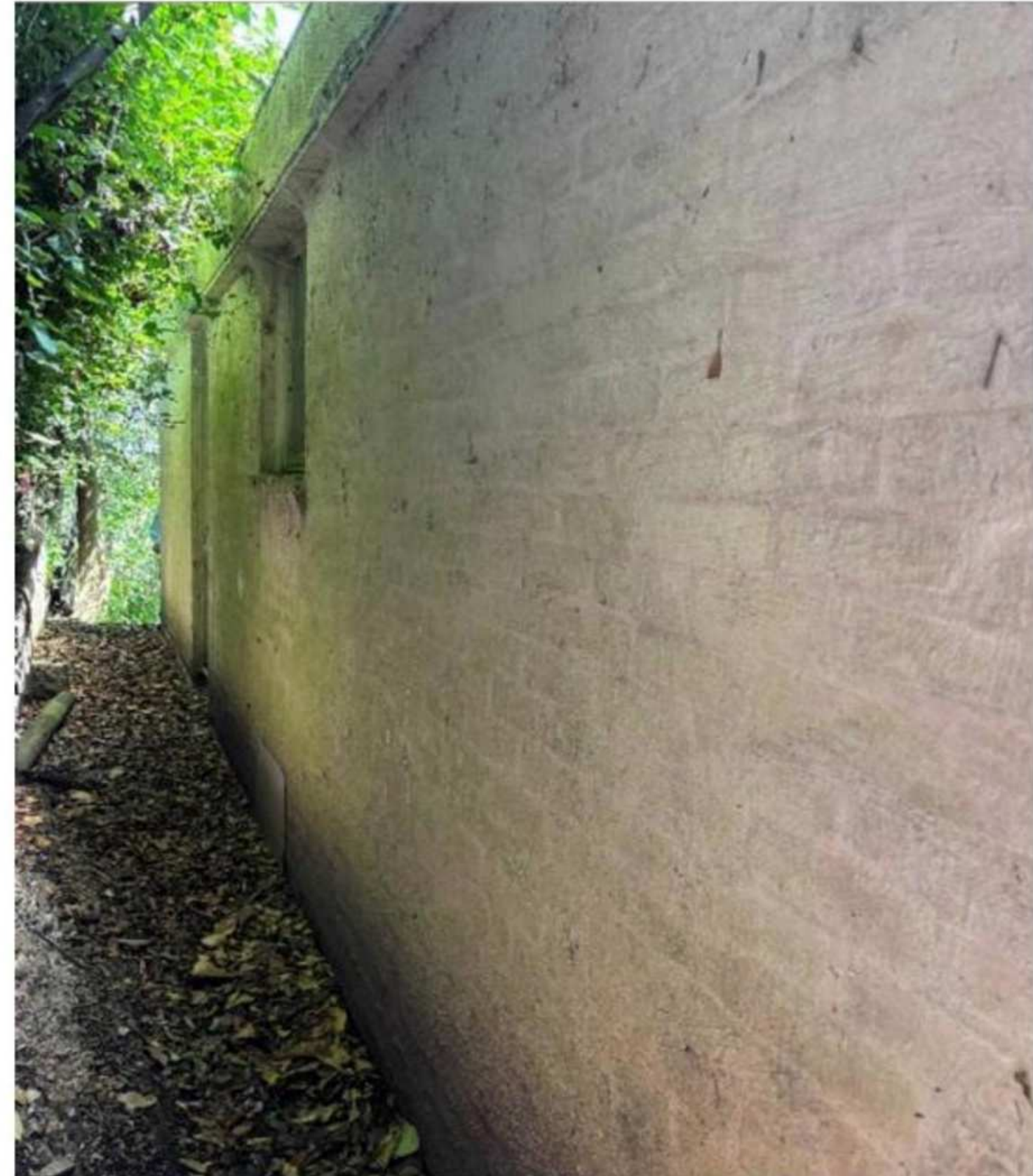
External walls on southern side
