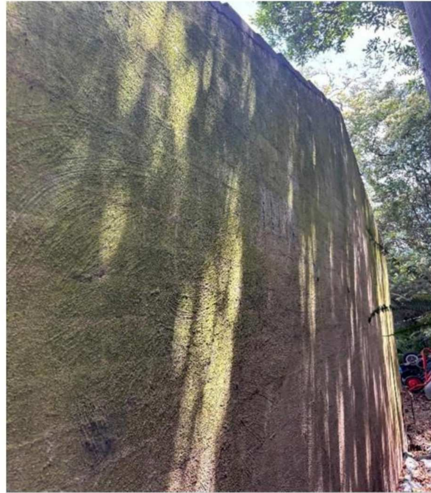
External walls on southern side
