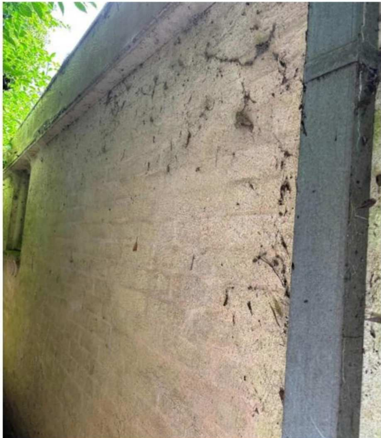
External walls on southern side
