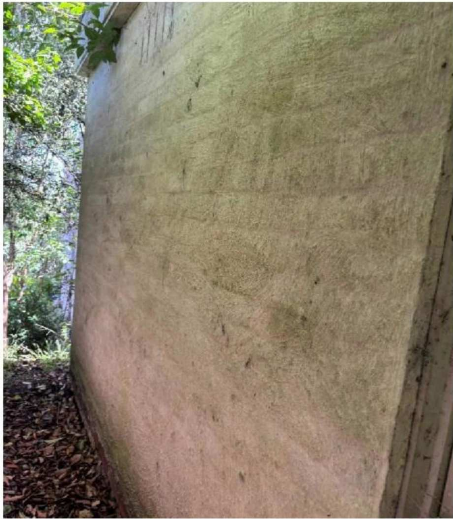
External walls on southern side
