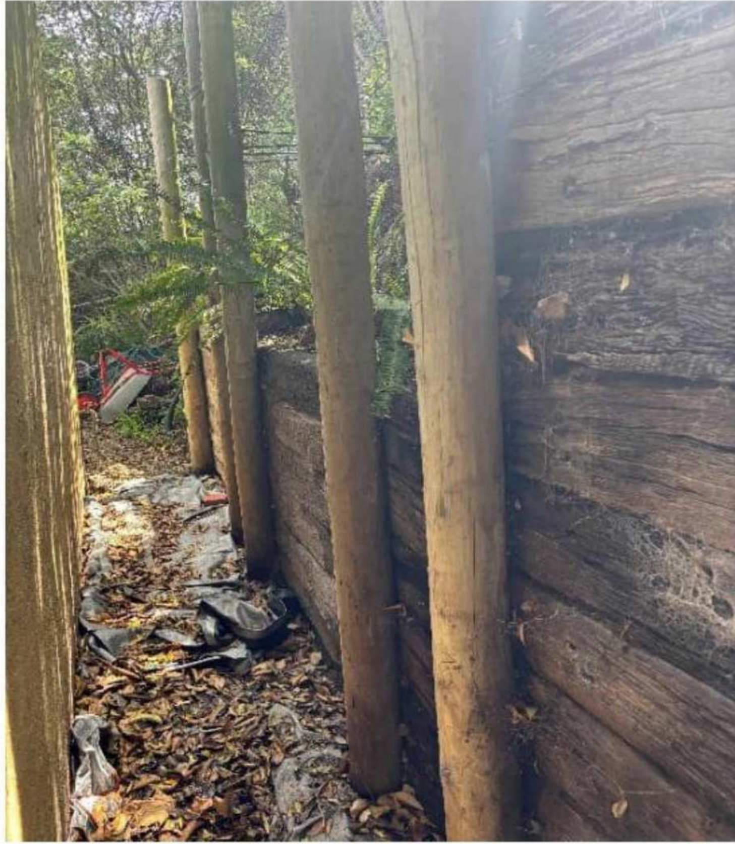
East side retaining wall
