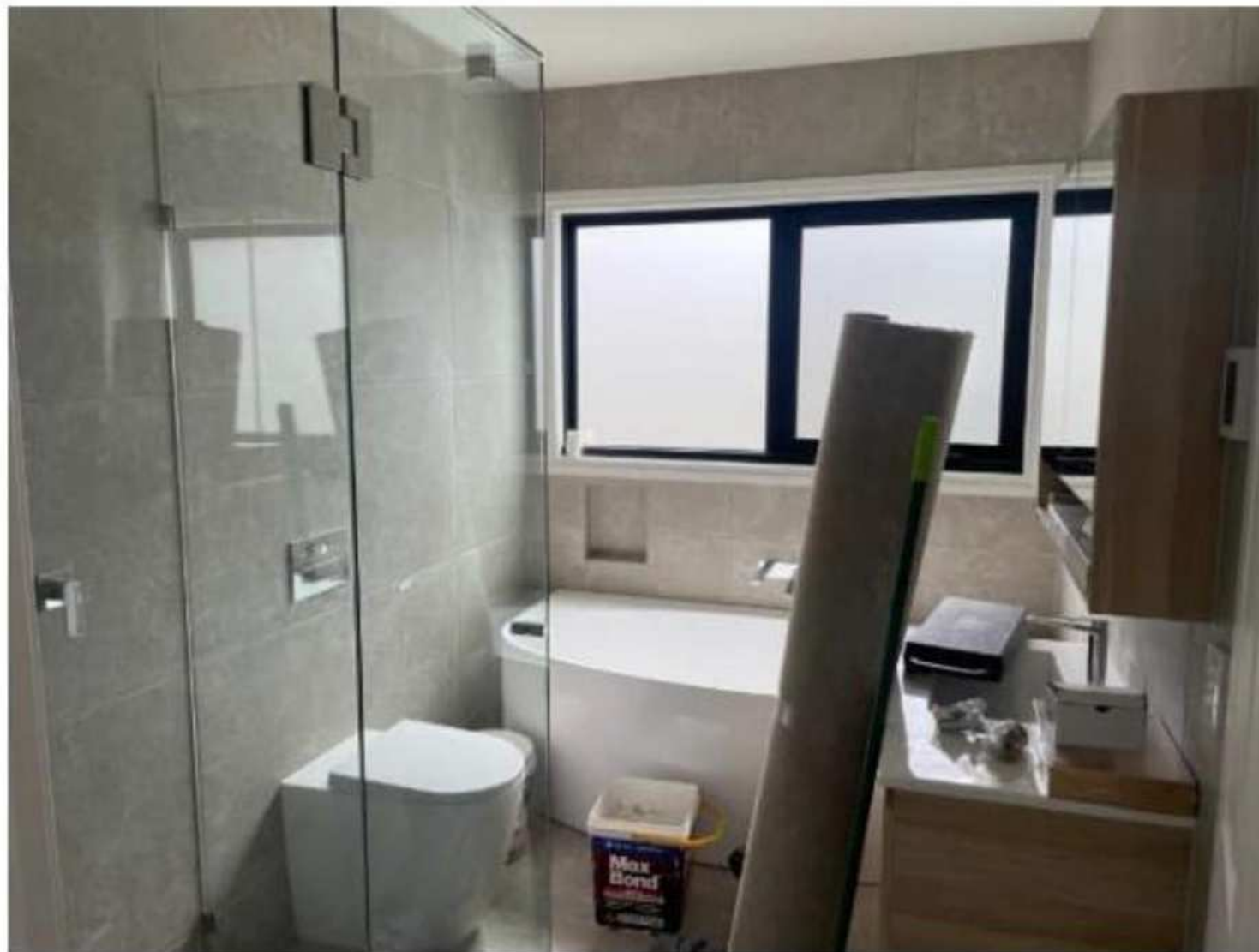
First Floor Bathroom
