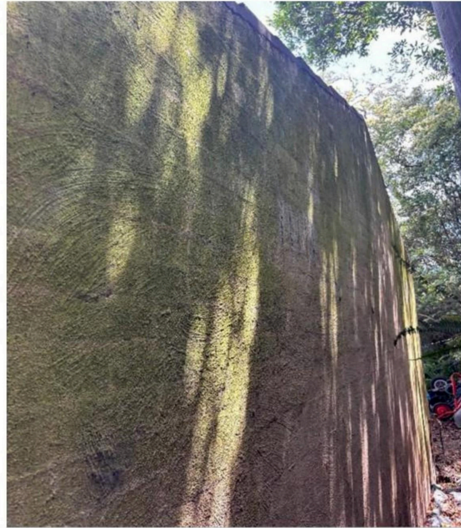
External walls on southern side
