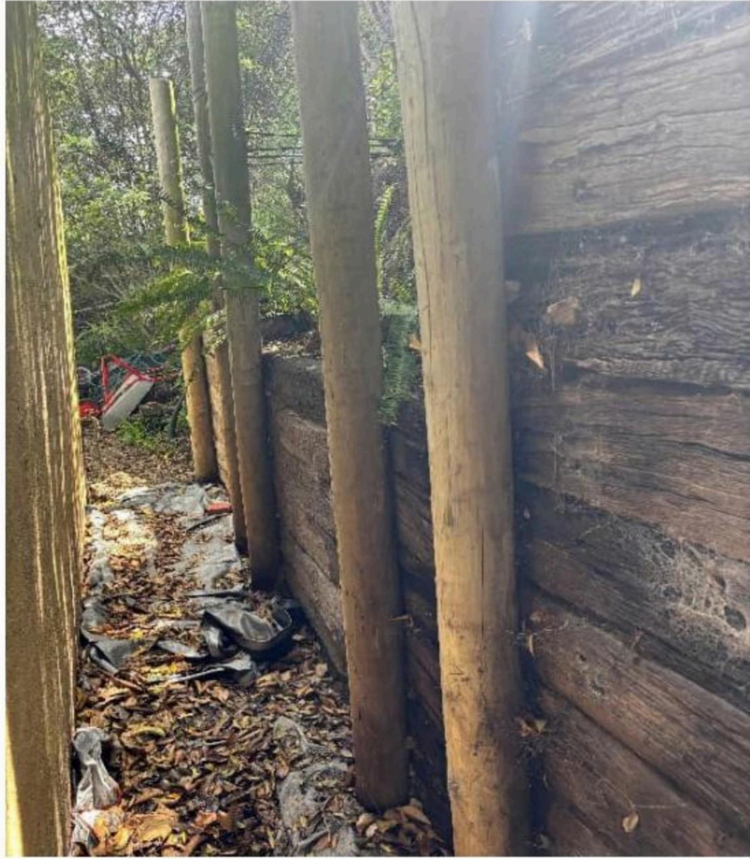
East side retaining wall
