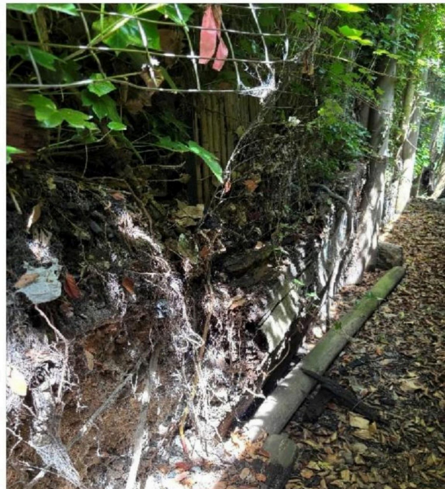
South side retaining wall
