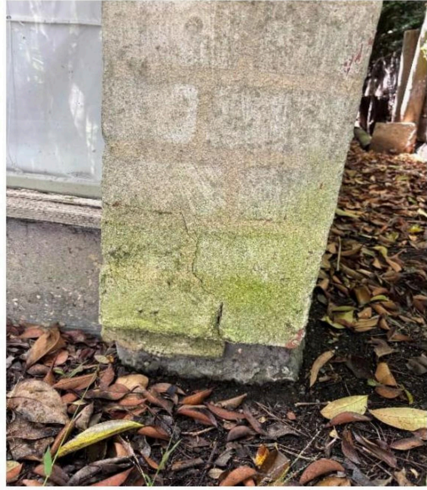
Wall on western side
