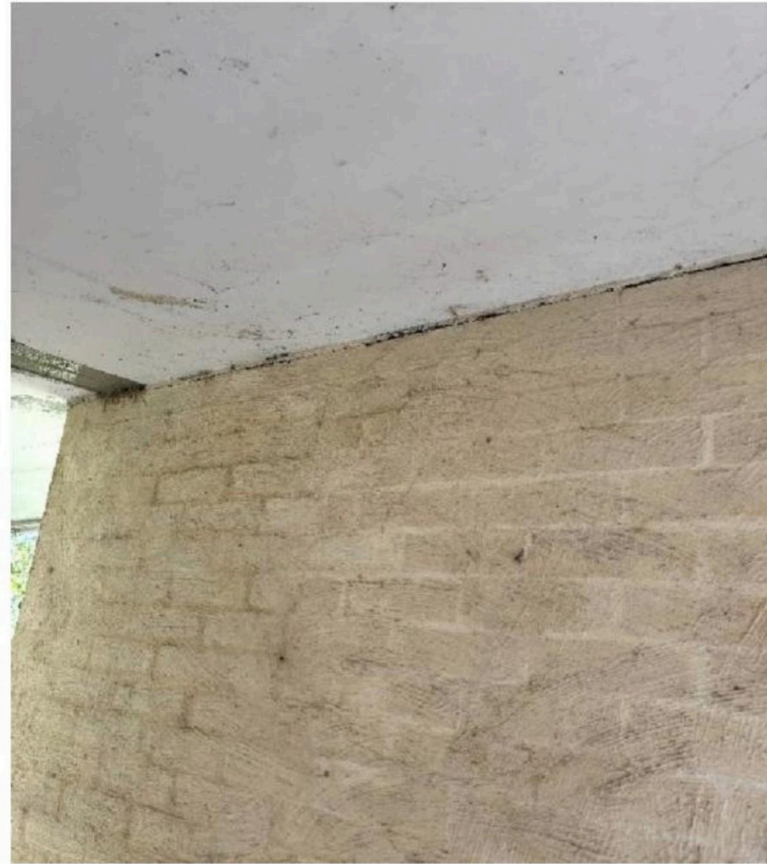
Eastern front wall
