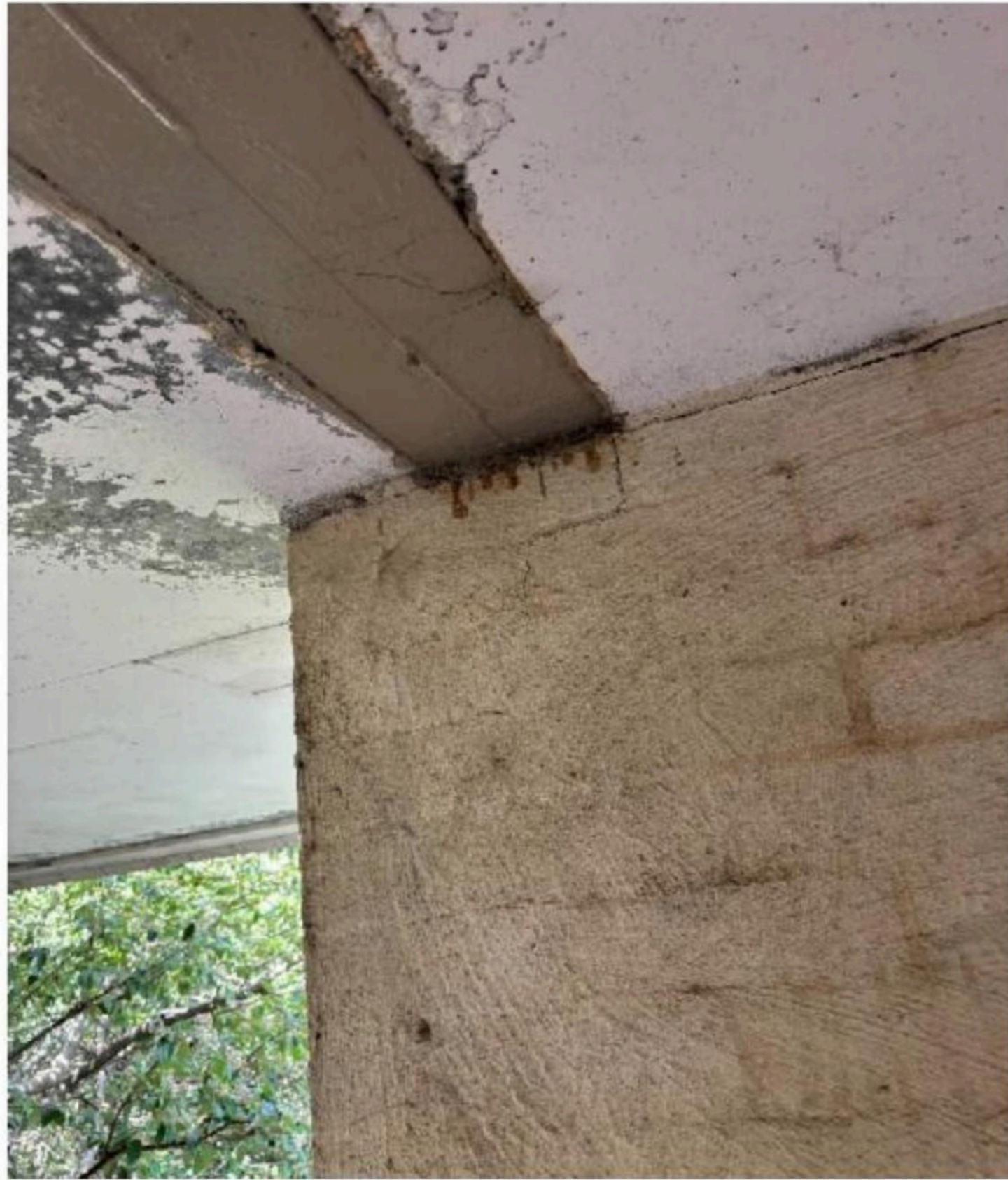
Eastern front wall
