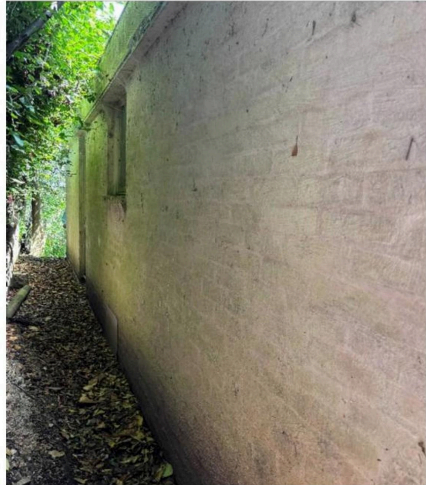
External walls on southern side
