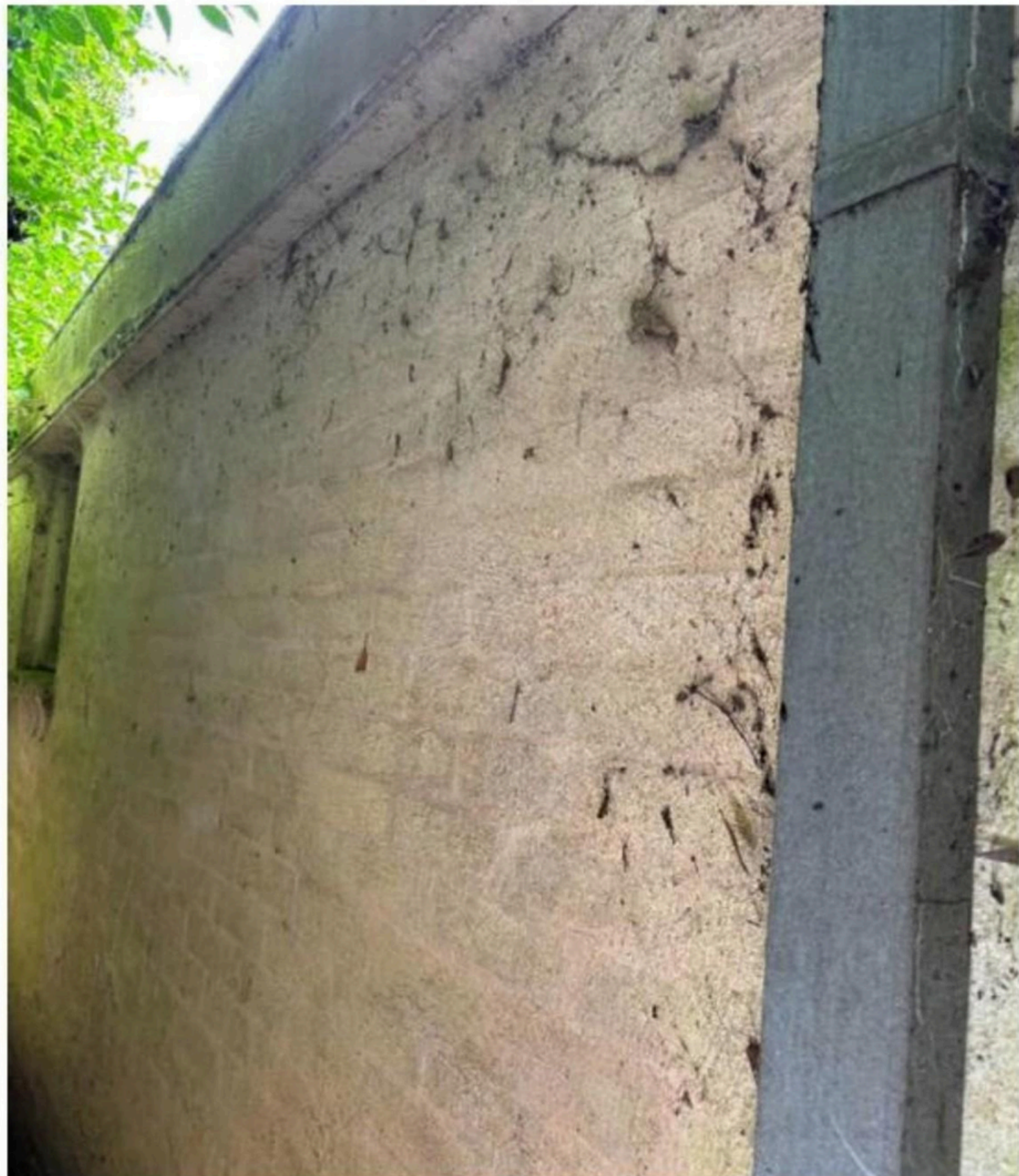
External walls on southern side
