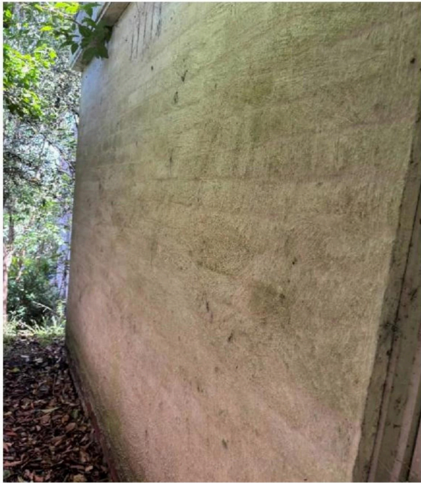
External walls on southern side
